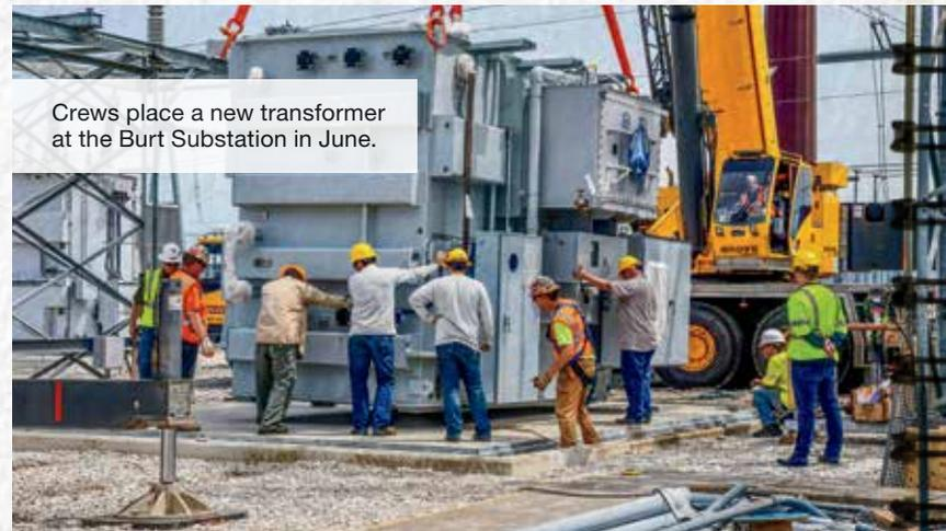
Crews place a new transformer at the Burt Substation in June.
