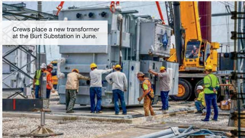
Crews place a new transformer at the Burt Substation in June.
